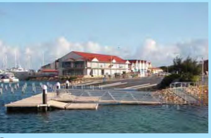
2 Universal Access Floating Pontoon Allows people with limited mobility to easily board and disembark from vessels. (See G6 on Inset Map A)
